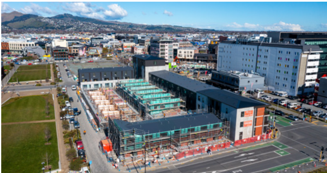
East Frame Residential Area, Christchurch
