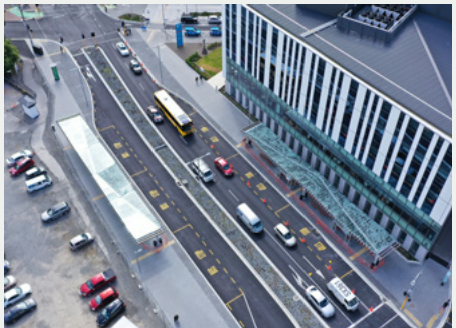
Tuam Street bus lanes and shelters, Christchurch
